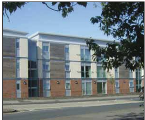
York Vale House development in Northallerton (Broadacres)
