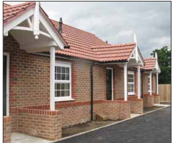
Oxmoor Place development at Easingwold (Yorkshire Housing)
